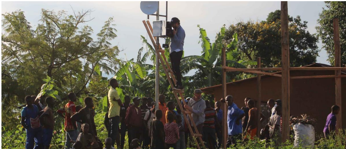
Set up of a node of the Wi-fi mesh at Idjwi. Photo courtesy Project First Light
