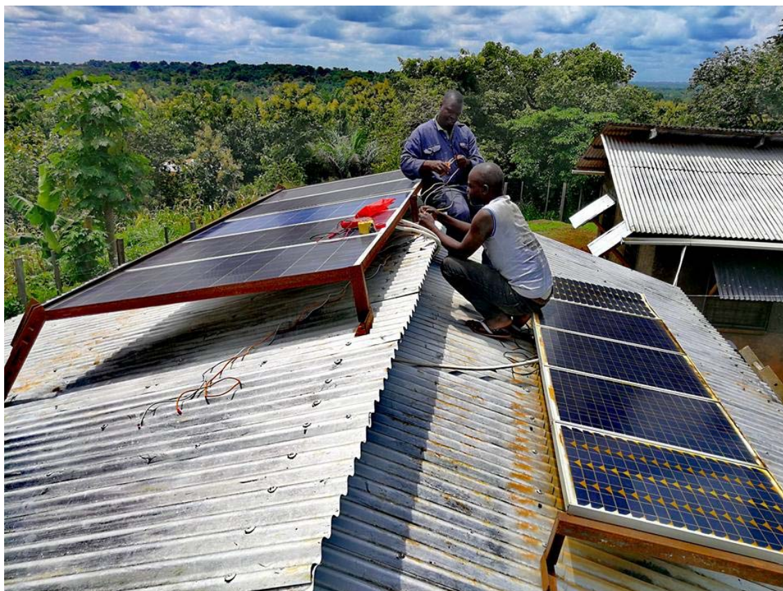
Vision net personnel setting up solar panels. Photo credit: Vision Net
